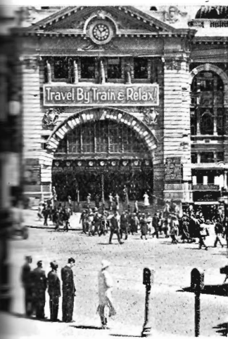
ADDITION TO the calico sign in this picture, a further sign is exhibited at the Elizabeth-st. entrance to Flinders-st. station. (Further reference in Page 2.)
